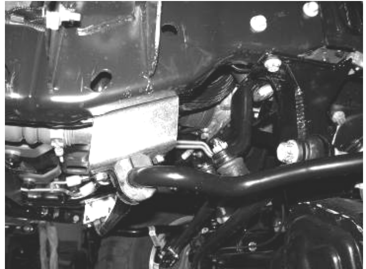
View of outer driver side frame rail
