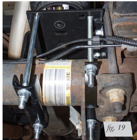
Right side (passenger) rearward axle view of finished installation torqued to 10ft. lbs.
