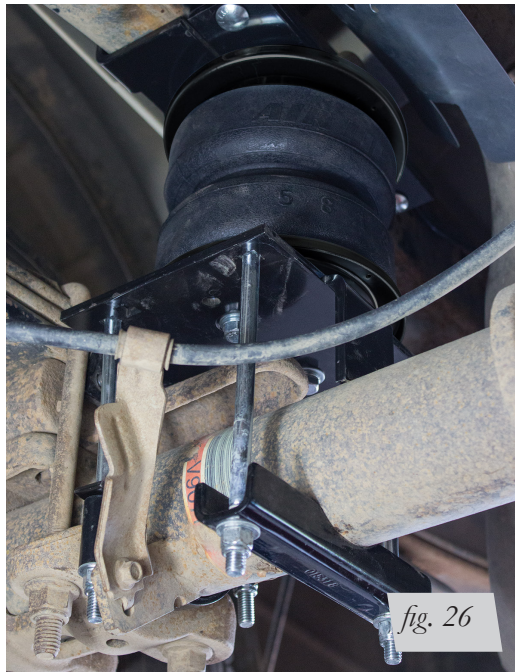
Right side (passenger): front view of installation.
