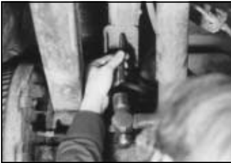
Center punch/drill out the rivets
