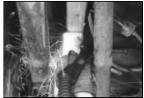
Cut off with a torch
