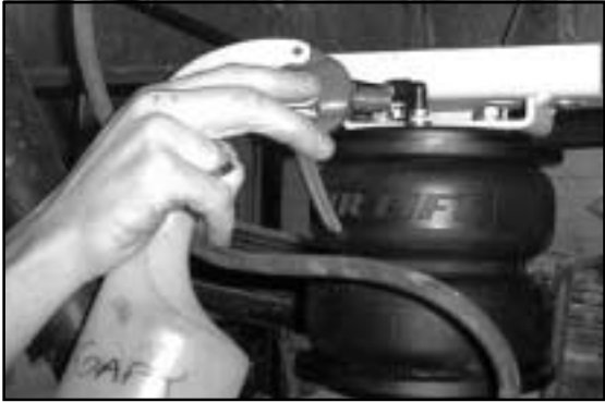
Leak test the air line connections and threaded connection of the elbow into the air spring. See page 12 to repair.
