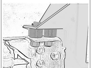
13. If necessary use the 25mm spacers provided in the fitting kit between the mounting bracket and the out riggers of the chassis. Fix in place with ½" x 2" bolts, ½" flat washers, ½" spring washers and ½" nuts. Do not tighten.
