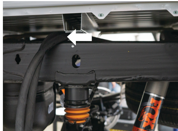
Fig. 36: Route the reservoir.
