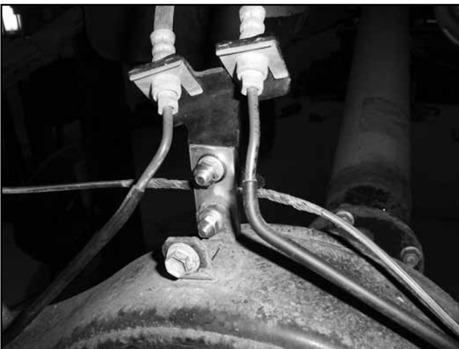
FIGURE 65A - LOOKING FROM BACK
