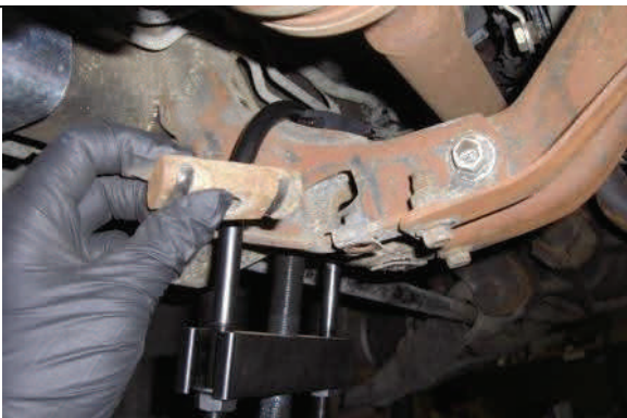
Adjust tool enough to remove keeper block
