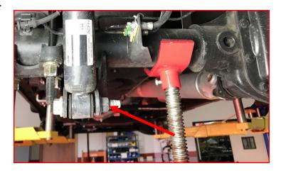
Loosen but do not remove the u-bolts on the passenger side. Completely remove the u-bolts on the driver side and discard. Lower the axle enough to install the ReadyLIFT block. Raise the axle while lining up the center pins on the axle and block. Install the provided u-bolts. Do not fully tighten at this time. Repeat for the other side of the vehicle.
