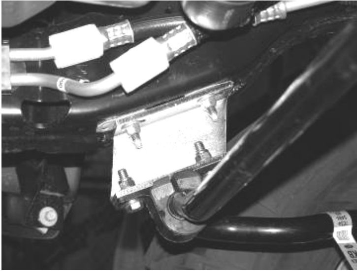
View of inner passenger side frame rail
